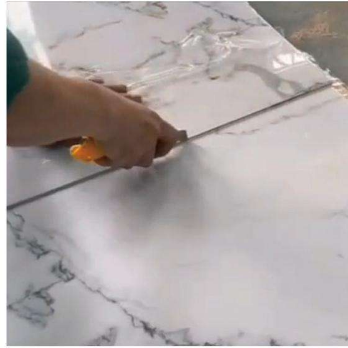
2.Cut the UV wall panel with a utility knife.
