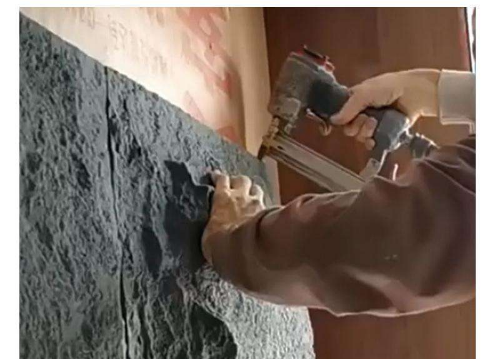
4.Nailing for Reinforcement
